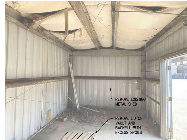
03 METAL SHED INTERIOR (VIEW LOOKING NORTHEAST) SCALE: N.T.S.
